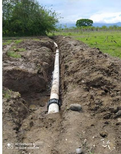
**DAÑO EN TUBERÍA DE 14" OCASIONADO CON RETROEXCAVADORA DURANTE
